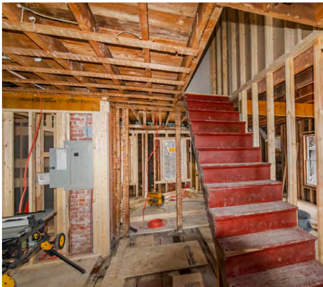
Renovations underway at Jonah Richard's multi-unit development project in Bradford, Vermont.
