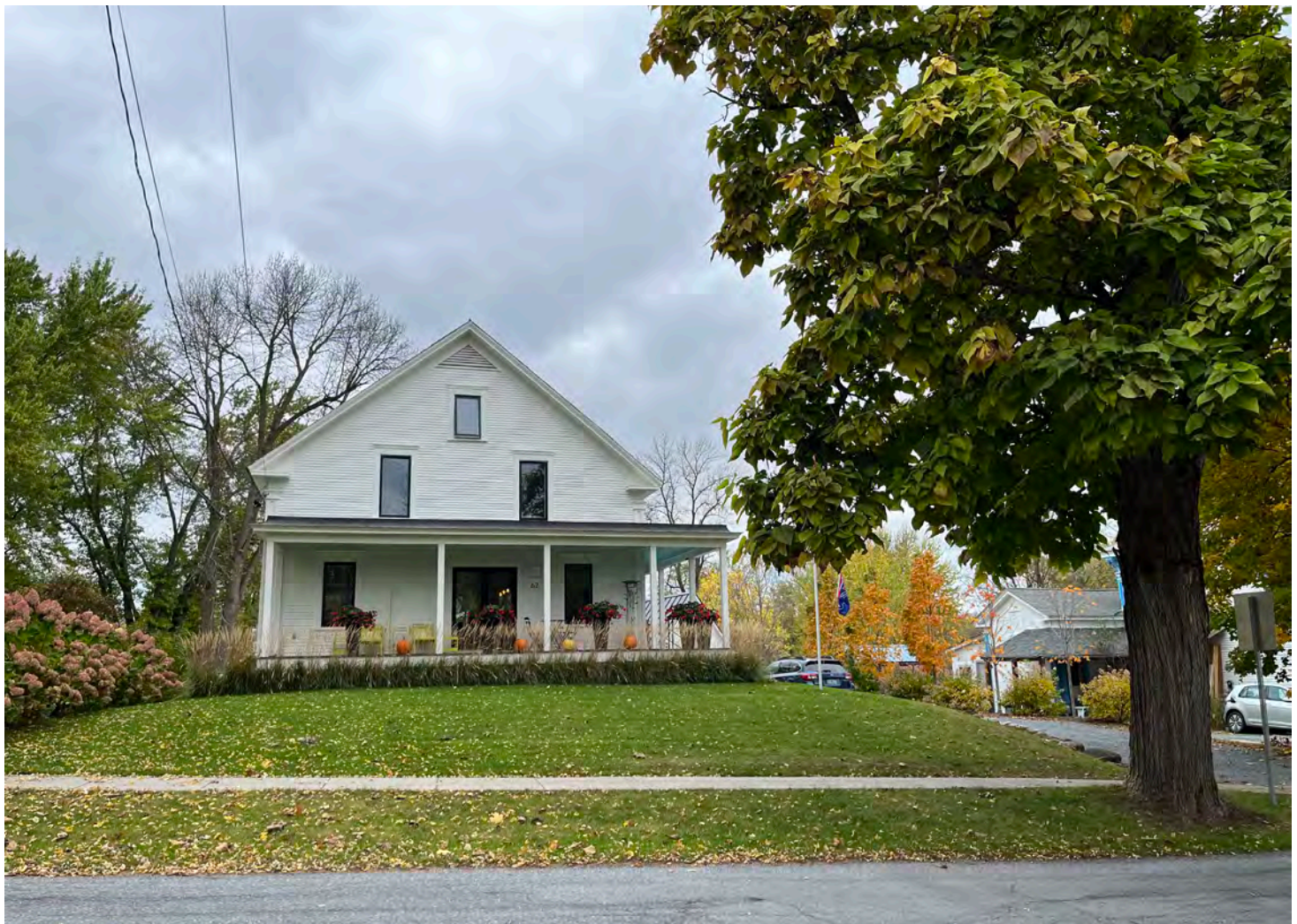
A recent renovation of a historic home in Vergennes, Vermont, showcasing the kind of investment that is possible when local officials are engaged in encouraging small-scale development and reinvestment through improved regulations and processes.
