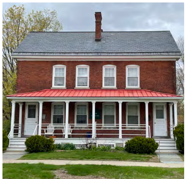
Existing side-by-side two unit home in Vermont.
