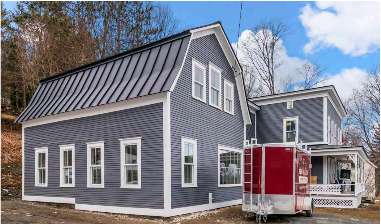
Finished exterior of Jonah Richard’s multi-unit renovation project in Bradford, Vermont.
