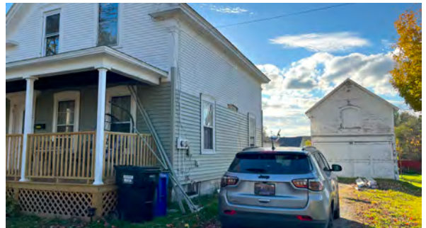
Potential attached and detached ADU conversion types for two existing Vermont homes.
